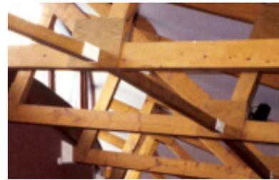
Poorly detailed connectors can prevent effective re-use of timber.
