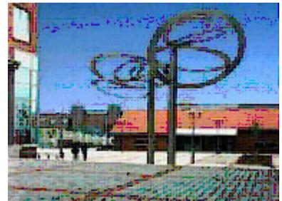
Concrete paviors can be re-used with sand bedding and allow access to services below.
