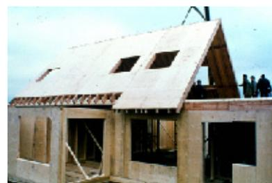
Pre-fabricated composite panelling structure.
