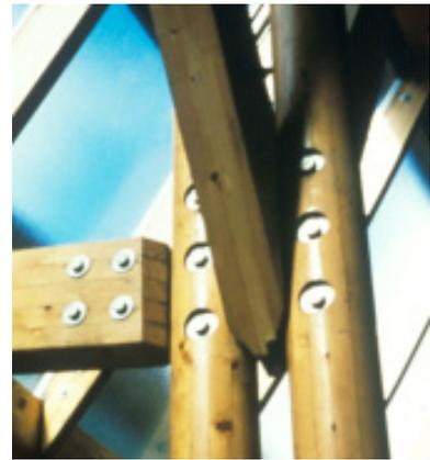
Try to minimise interpenetration of connectors with components.
