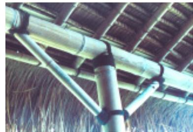
Friction jointing is the least disruptive form of fixing.
